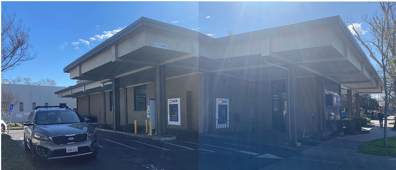
North façade with covered driveway, composite view facing southeast. Source: ESA, 2024.
